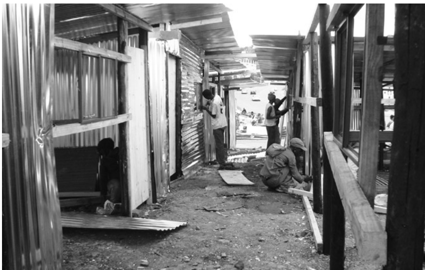
▼ Figure 4: Realigning shacks - Quarry Road, Durban. Photo: Samke Phewa, CORC
