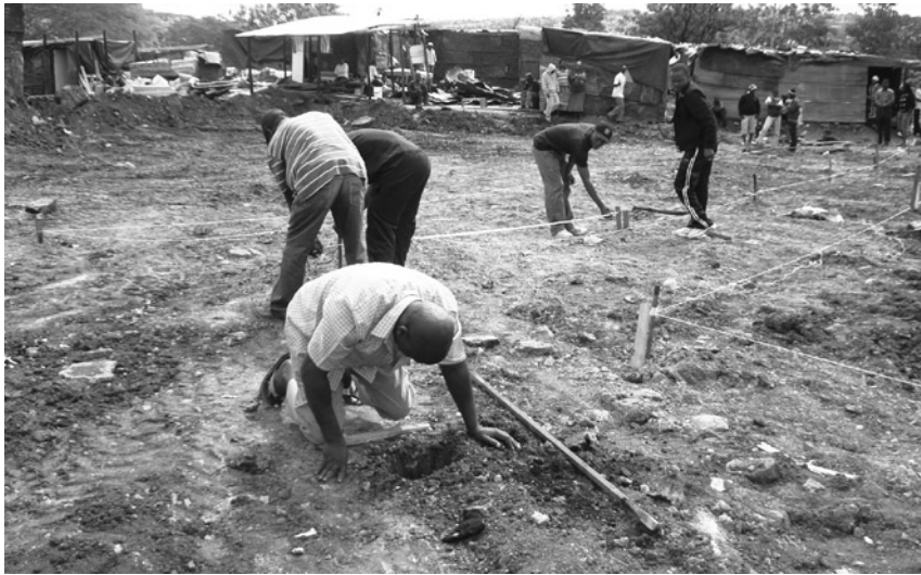
▲ Figure 3: Pegging out sites: Quarry Road, Durban. Photo: Samke Phewa, CORC
