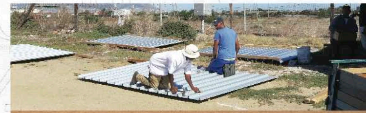
iKhayalami during construction in Kuku Town, Cape Town April 2014
